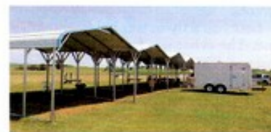
Nice shelters are available at Farview for pilots to keep equipment cool and dry in the unpredictable summer weather.
